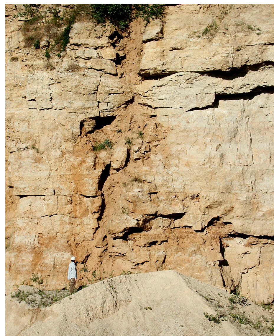
Bedrock cavities —This exposure in a quarry wall is an example of the cavities in Prairie du Chien Group bedrock that partially filled with unconsolidated sand, silt, and clay, and are likely present beneath many sinkholes. Surface water carried unconsolidated surficial deposits into the cavities.
